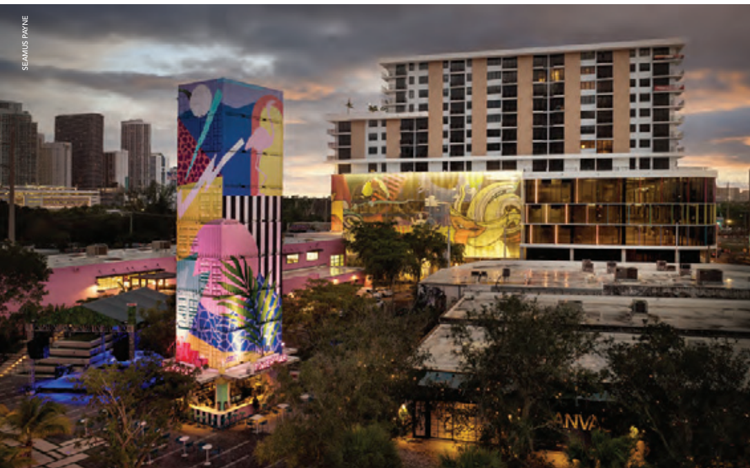
Strata Wynwood, an eight-story, mixed-use structure, added 257 studio and one- to three-bedroom rentals (509 to 1,288 sf), 2,500 sf of artist studios, and three floors of office space to Miami’s Wynwood Arts District. Stantec (architect, SE, landscape architect) helmed the project team of Unison Group (interiors), Feller Engineering (MEP/FP), and KAST Construction (GC).
