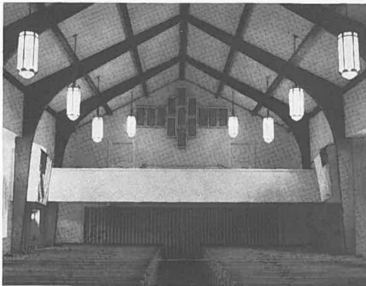
Attractive arrangement of sound panels projects antiphonal organ from rear gallery wall at the Church of the Nativity, Buffalo, New York (no organ chamber).
