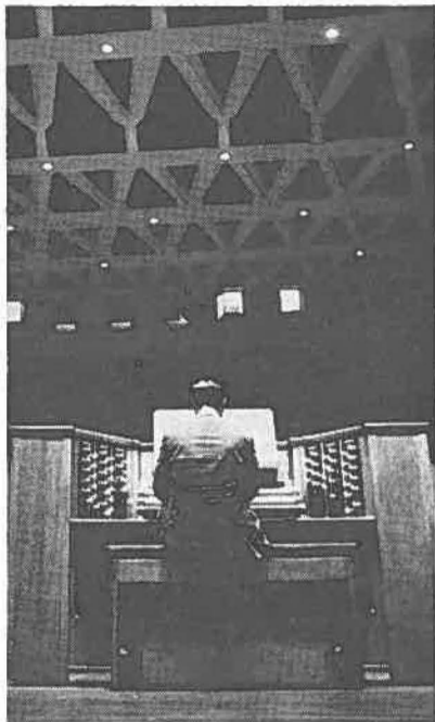
This view shows the console, which though large can be seen over; and the striking ceiling frame which regulates the lighting and has some control over the acoustics.
