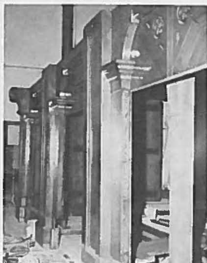
Newly oiled casework.
