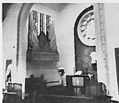
Wicks Organ Co. of Highland, IL, has built a 2-manual and pedal organ of 7-ranks for Zion Lutheran Church, Elgin, IL. The instrument is in an existing chamber, with Great pipes exposed in front; the installation and tonal finishing was by Russell Joseph-Daniel Bogue Associates.
