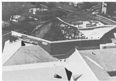
View of auditorium roof
