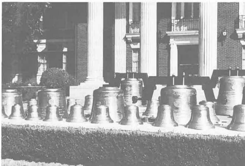
Bells of the Baylor Carillon before installation
