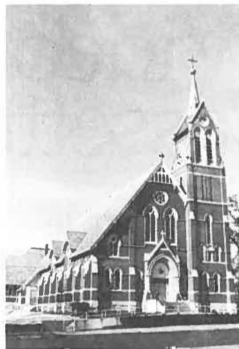
St. Simon Catholic Washington, IN 3 Manuals — 53 Ranks Completion 1989
