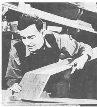
William Dowd in the Hubbard & Dowd shop, notching the corners of a harpsichord case to insert splines or keys to strengthen the joints.
