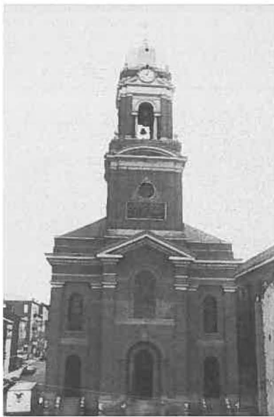
St. Paul's, Cincinnati, presently Verdin's Corporate Headquarters and the Verdin Clock and Bell Museum.
